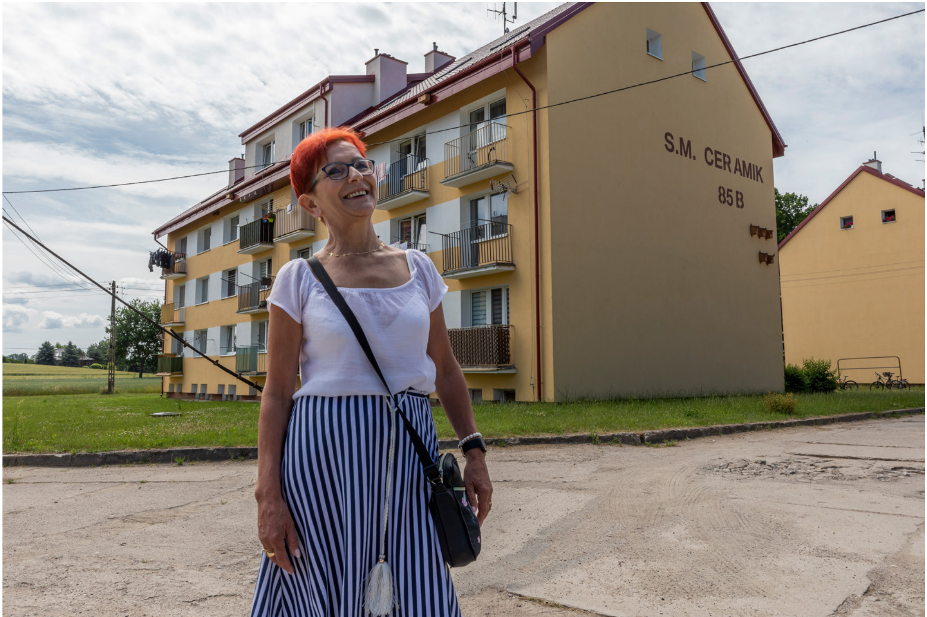
Ceglowo, Poland - Bozena Wasiak, a resident of the Soviet-era Ceramik housing units that have been regenerated with photovoltaic panels and heat pump systems.
