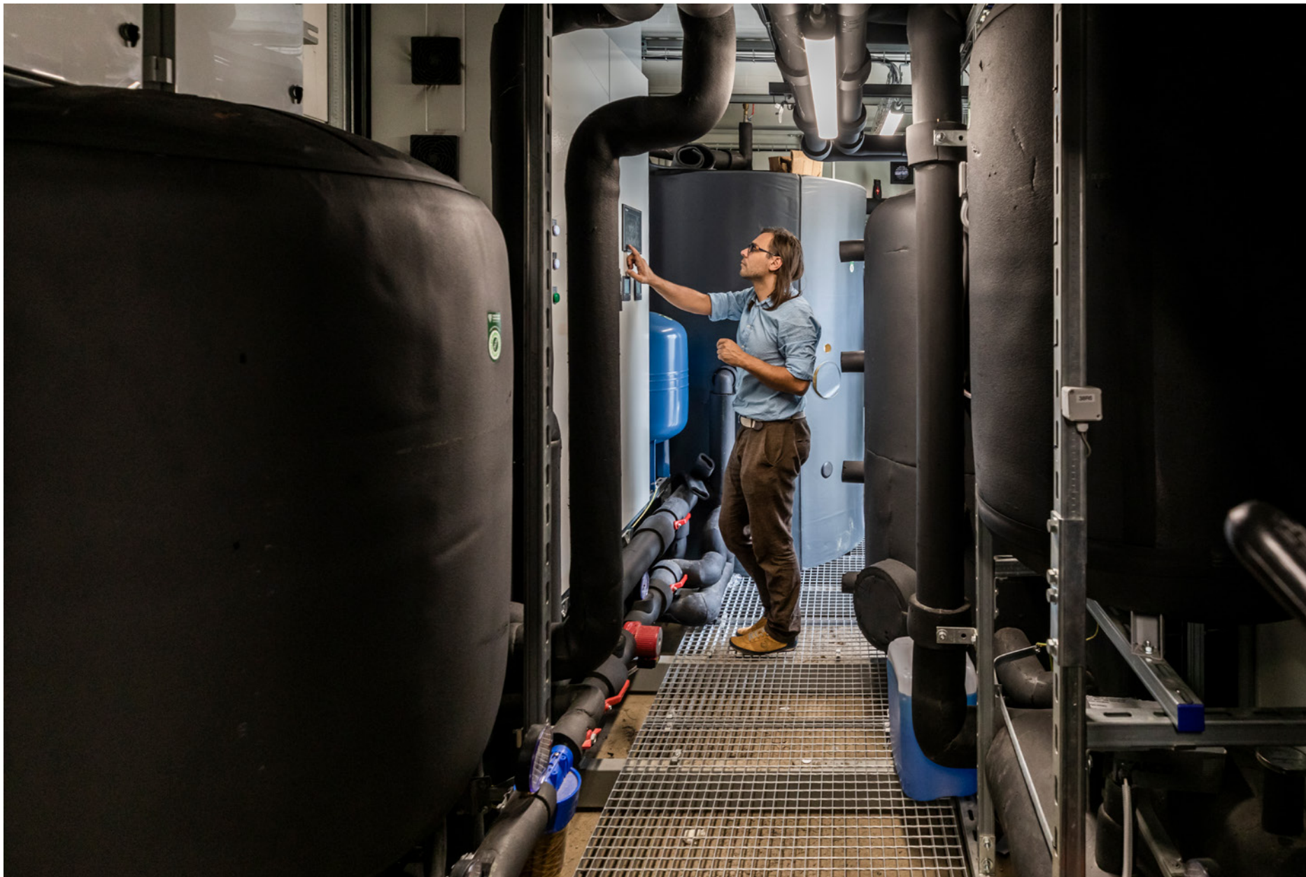
Zwolén, Poland - Kamil Kwiatkowski, director of research projects for the Euros Group, checks the heat pumps in one of the Soviet-era housing units that have been regenerated with photovoltaic panels and heat pump systems.
