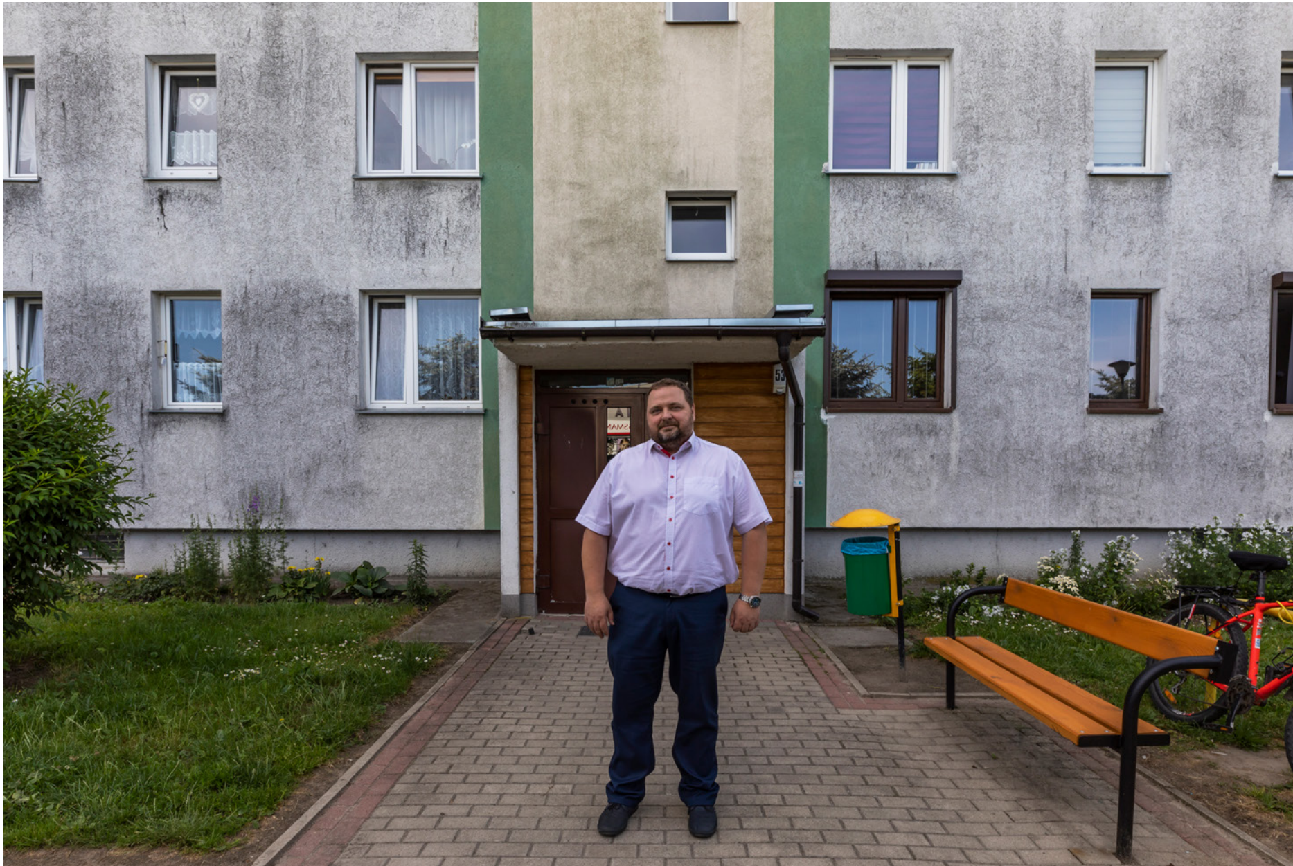
Bartoszyce, Poland - Wojciech Sienkiewicz (45), president of a group of Soviet-era housing units that have begun the process of ecological renovation with photovoltaic panels and heat pump systems.
